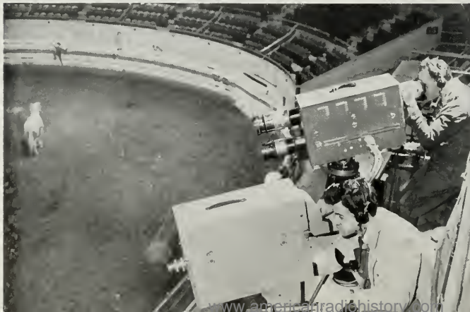
NBC ANNOUNCER BEN GRAUER AND USHERETTE BETTY BEUHLER DEMONSTRATE HIGH SENSITIVITY OF IMAGE ORTHICON USING ILLUMINATION OF ONE CANDLE. BELOW: GREATLY SUPERIOR SENSITIVITY OF CAMERA USING THE IMAGE ORTHICON (FOREGROUND) IS COMPARED WITH PERFORMANCE OF CONVENTIONAL CAMERA IN PICKING UP SCENES FROM THE RODEO AT MADISON SQUARE GARDEN.
