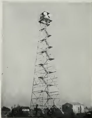
AUTOMATIC, UNATTENDED RADIO RELAY TOWERS, LIKE THE ONE ABOVE, MAY ULTIMATELY REPLACE THOUSANDS OF MILES OF TELEGRAPH AND TELEPHONE LINES IN THE UNITED STATES.
