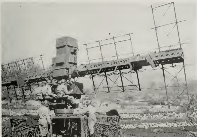
EARLY MODEL OF RADAR IN OPERATION ON AN ITALIAN HILLSIDE. THE THREE GRID-LIKE ANTENNAS GIVE AZIMUTH, ELEVATION AND RANGE OF OBJECT DETECTED.
