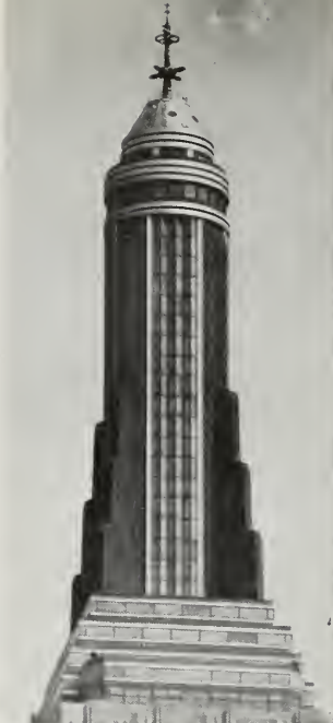
ELEMENTS OF THE NEW ANTENNA ARE VISIBLE ATOP THE CIRCULAR PORTION OF WNBC'S TELEVISION ANTENNA.
